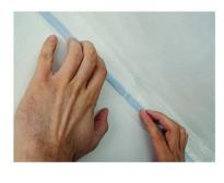
Press vapour barrier firmly onto the OTTOCOLL® A270 bead
