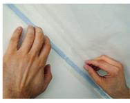
Vapour retarder has to be applied with loop to compensate movements
