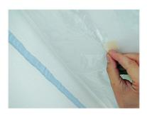
Fix vapour retarder with adhesive tape. Apply OTTOCOLL® A 270 in a bead of 8 mm and leave to set for 1 - 3 days
