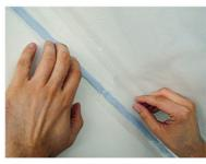
Apply vapour barrier with loop in order to compensate movements of the building.
