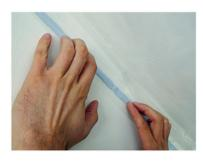
Press vapour barrier lightly onto the bead CAUTION:
