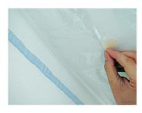
Fix vapour barrier in place with adhesive tape. Remove the fixed vapour barrier immediately after applying OTTOCOLL® A 270 in 8 mm beads.
