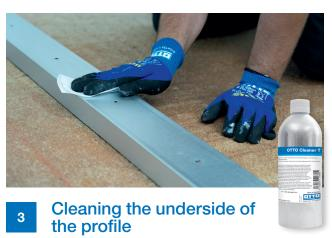
Cut the profile to length, place it next to the marking with the adhesive surface facing upwards and clean thoroughly with OTTO Cleaner T.
