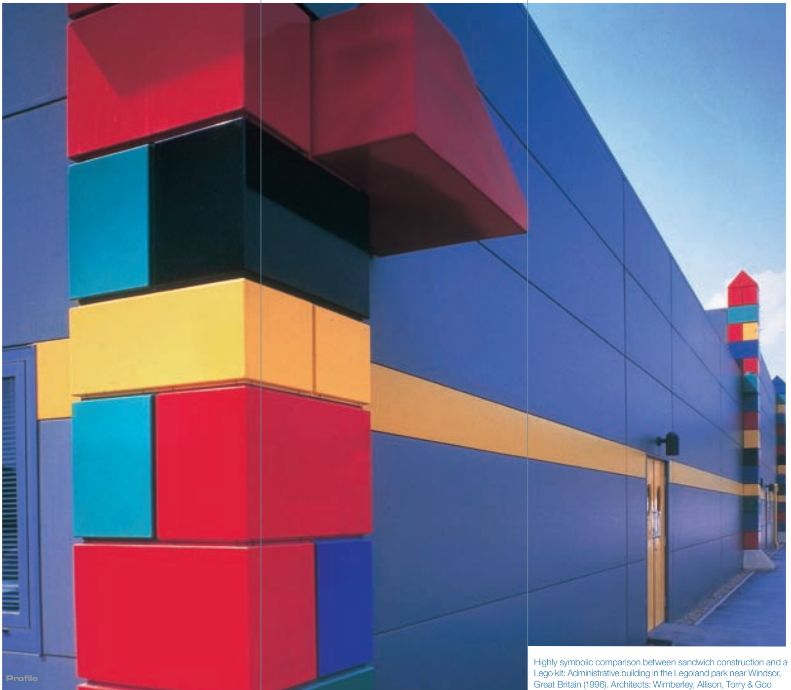
Foamed layers of a sandwich element provide load-bearing properties and inherent stiffness by means of the shear strength of the bond between the insulating core and the outer layers.
