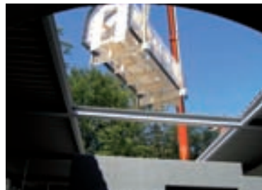
A low-platform trailer places the preassembled segments in the concrete foundation.
