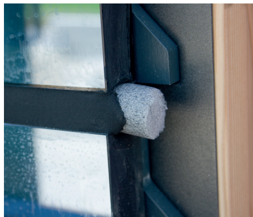
Sealing with sealant and PE back-up foam rod
