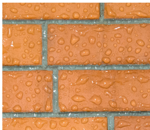
Façade with hydrophobic treatment using OTTO Siloxan 290L
