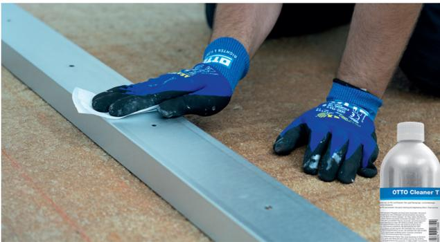
**3 Cleaning the underside of the profile**
