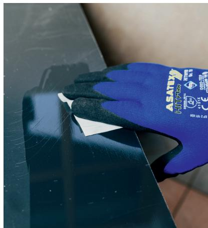
The load-bearing capacity of the substrate is a prerequisite for the bonding of OTTOCOLL® M 595. For absorbent substrates such as cellular concrete, a load-bearing capacity can be achieved by pre-treating with OTTOFLEX Deep Primer. In sanitary areas, direct bonding onto OTTOFLEX Protective Coating is possible. The basic prerequisite for good adhesion is to ensure that the material substrates to be bonded are grease and dust-free, which can be accomplished with a cleaner such as OTTO Cleaner T.
