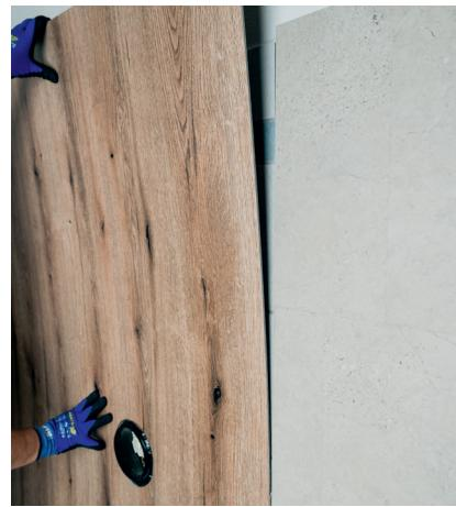
Before attaching the wall cladding panel, the adhesive must first be moistened. This step is not required if a slightly moist, absorbent (but touch-dry) substrate is being used.
