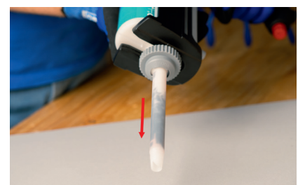
Fill the static mixing nozzle with adhesive. Check the homogeneity of the mixture (see the quality checks for 2-component products to be carried out during processing)
