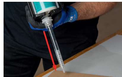
Fill the static mixing nozzle with adhesive. Check the homogeneity of the mixture (see the quality checks for 2-component products to be carried out during processing)
