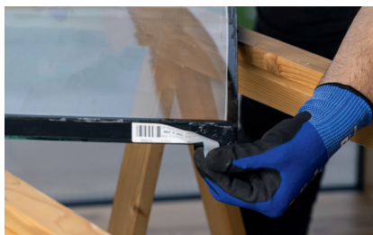
Remove stickers from the insulating glass
