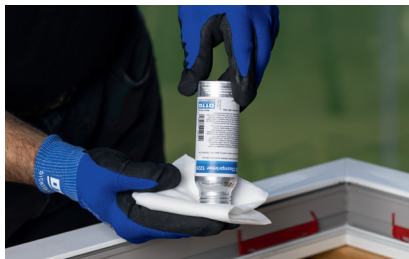
Wet the cloth with OTTO Cleanprimer (or Cleaner + Primer) 1)
