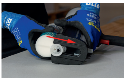
Insert the side-by-side cartridge into the gun
