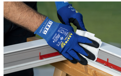
Pre-treat the profile's adhesive surface with OTTO Cleanprimer (or Cleaner + Primer) 1)
