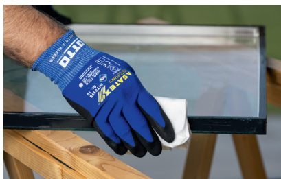
Clean the edge sealant with OTTO Cleanprimer (or Cleaner + Primer) 1) and a fabric cloth
