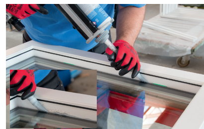
Fill the rebate base with adhesive
